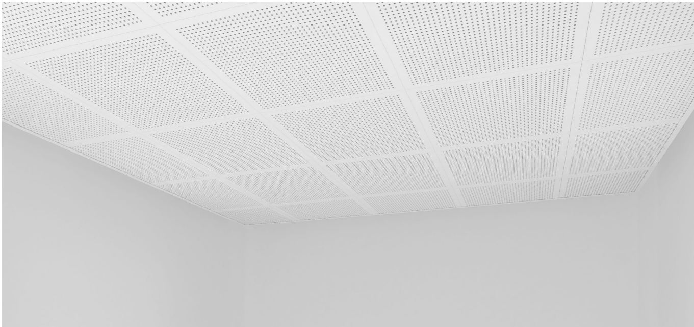
12 Individually demount each tile in this system for maintenance. To remove any tile, slightly raise the tiles on one side until they can be slid off the main profile.
