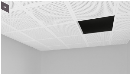
12 Individually demount each tile in this system for maintenance. To remove any tile, slightly raise the tiles on one side until they can be slid off the main profile.
