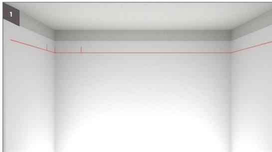
1 Use a laser beam to measure and plan the ceiling layout in advance so that the tiles adjacent to the walls are not less than 300mm width
