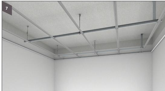
Connect the spring tee to the primary channel at 600 spacing using wire connecting clip WCC
