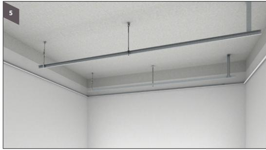
Fix the primary channel at 1200 mm spacing
