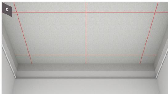
3 Mark with laser the hanger spacing at 1200 mm o.c.
