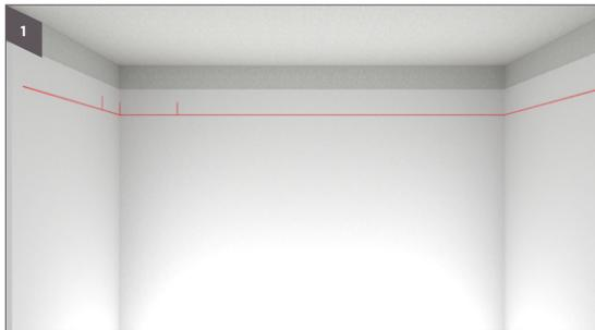
1 Use a laser beam to measure and plan the ceiling installation process where the min distance of Spring tee shall be 300 mm and shall not exceed 450 mm from wall
