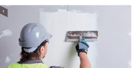
**Step 1**Finishing coat for square edge joints
