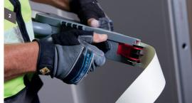
Adjust the nozzle to ensure at least 1mm of compound is in under the tape
