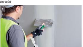
For second and finishing coats apply as per tapered or square edge joint and finishing application
