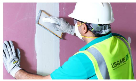
Application of joint compound over tapered edge joint
