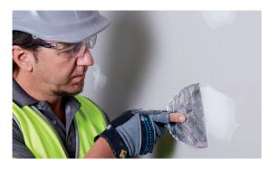
Applying 3 separate coats of joint compound over screw fixings
