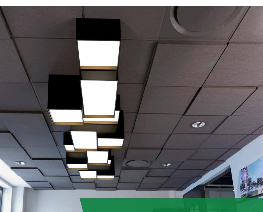
In administration offices avoid direct sound pathways between cubicles and offices by proper placement of wall partitions and ceilings tiles. Open office and general administration office should be designed to provide an acceptable level of speech privacy between adjacent offices. 50 dB wall partition assembly can achieve the General Administration Offices requirements, and mineral fiber ceiling as Sonata tiles will be necessary to control the reverberation time.
