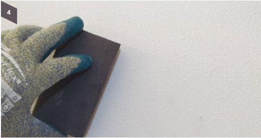
Step 2 Try lightly sanding the soiled area with a sanding sponge such as a very fine grade sanding hand pad
