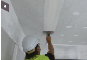
Step 6 Apply final coat
