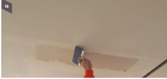
Step 16 Feather out joints flat from the new patch and the existing ceiling using USG ME Finishing Compounds
