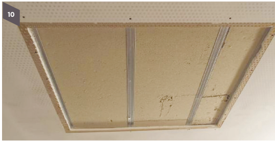
Step 10 Cut new acoustical backer panels to size and insert them where needed
