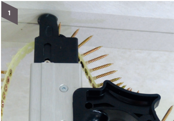
Step 1 Using a collated screw gun, screw fix the recessed & butt joints at 150mm centers
