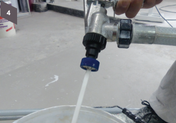
Step 4 Four coats of MAC plaster spray applied finish must be applied
