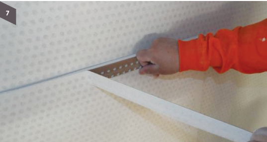
Step 7 After the new panel is cut to size, score the paper and veil 40mm from the perimeter, to make room for the tape on the joint
