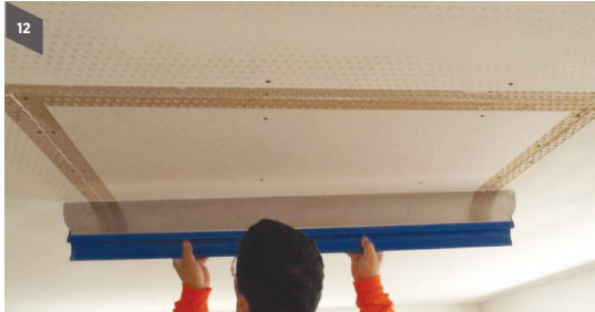
Step 12 Use a long straight edge to make sure the new panel is flush with the existing ceiling
