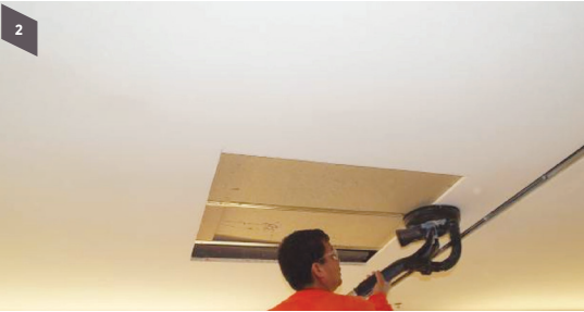
Step 2 Sand the existing coating off, down to the front veil, on the board around the entire perimeter of the area to be patched
