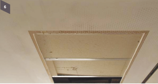
Step 6 Repeat this on all the sides of the area to be patched
