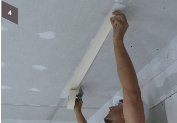
Step 4 Fill in the joints with Monosilent compound
