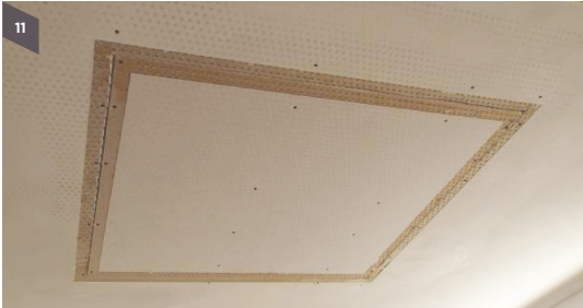
Step 11 Install the replacement panel, and be sure to insert additional screws around the perimeter of the existing ceiling at 150mm centres
