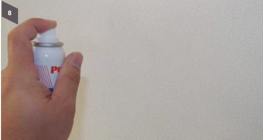
Step 7 Once the spray is coming out consistently, lightly coat the soiled area in a cross-hatch pattern. Hold the tip 30 to 35cm away from the target. Allow ample time to dry between coats. Circulating the air by using fans can significantly help decrease dry time
