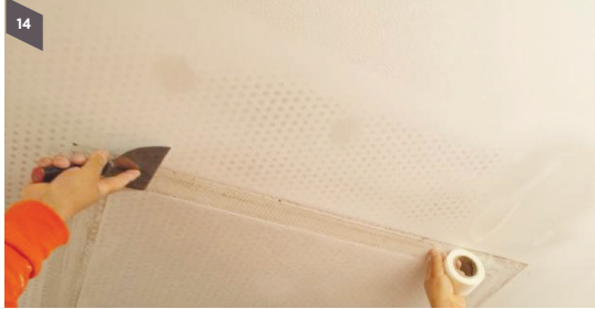
Step 14 Use USG ME or Sheetrock® branded paper or mesh tape or equivalent on all joints
