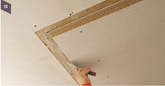
Step 13 Pre-fill all the gaps as tightly as possible with USG ME Joint Compound. Spot all screws with USG ME Joint Compound
