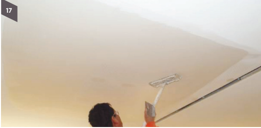
Step 17 Sand all the joints level/flat with the existing ceiling
