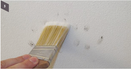
Step 1 Try to brush the soiled area with a soft brush such as a 5cm nylon bristly paint brush
