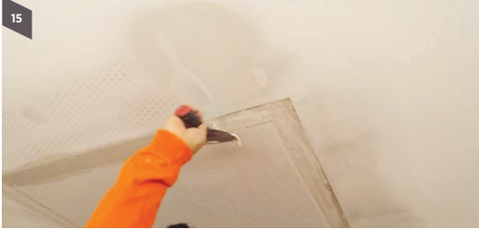
Step 15 Fill all joints and spot all screws with USG ME Joint Compound
