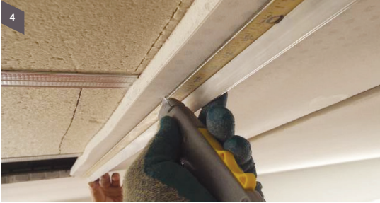
Step 4 Score the veil and paper 40mm from the edge around the area to be patched
