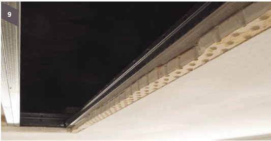
Step 9 Add additional framing as needed to support the new boards
