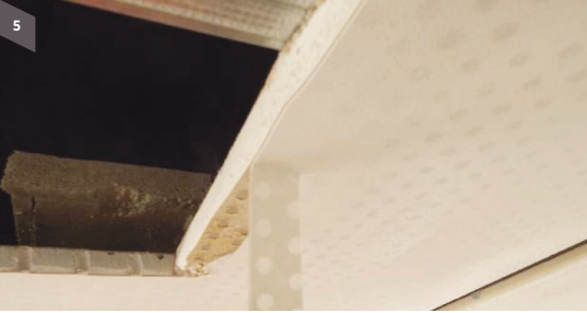
Step 5 Peel off the paper and veil to create room for the tape
