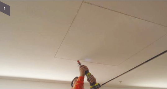
Step 1 Remove the affected area of the ceiling. Make all cuts as straight as possible so the new boards will fit tight to the existing boards
