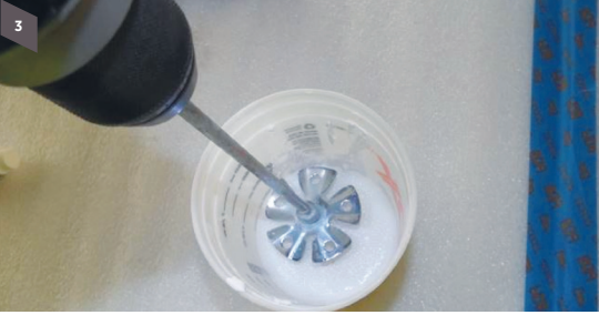
Step 2 Mix well with a drill and mixing blade
