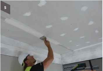
Step 5 Apply second coat
