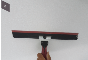
Step 6 Use soft rubber-bladed squeegee to remove any minor irregularities
