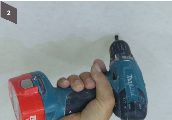
Step 2 Install screws Min. 30mm
