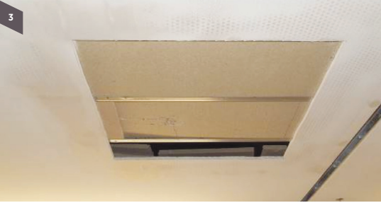
Step 3 Sand at least 400mm wider than the area to be patched
