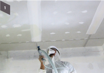
Step 1 Apply MAC plaster spray applied finish
