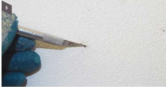
Step 3 For deep soiling, use a utility knife to lightly scrape away the soiled areas
