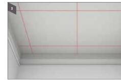
Mark with laser the hanger spacing at 1200 mm o.c.
