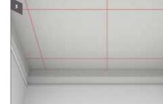
Mark with laser the hanger spacing at 1200 mm o.c.
