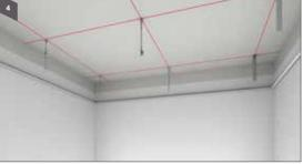
Fix hangers at 1200 mm o.c in a gradient scheme above the lines of primary channels
