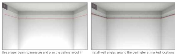
Use a laser beam to measure and plan the ceiling layout in advance so that the tiles adjacent to the walls are not less than 300mm width
