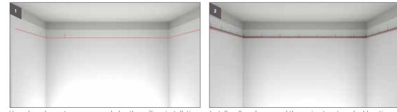
Use a laser beam to measure and plan the ceiling installation process where the min distance of Spring tee shall be 300 mm and shall not exceed 450 mm from wall
