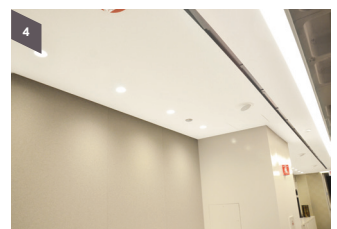
Step 4 Leave the ceiling to dry for a minimum of 24 hours
