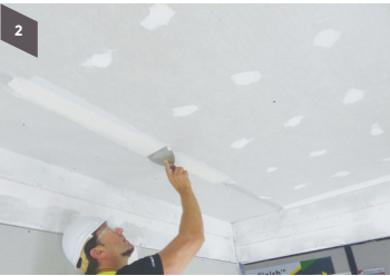
Step 2 Apply second coat
