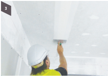
Step 3 Apply final coat
