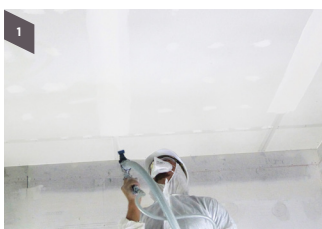
Step 1 Apply Monosilent Spray Applied Finish
