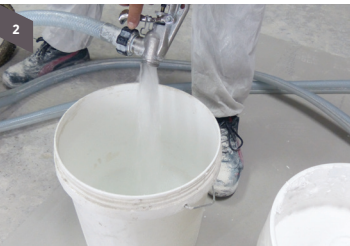
Step 2 Cycle water through the hose
