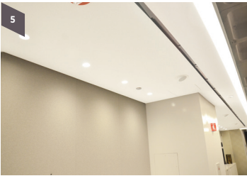
Step 5 Leave the ceiling to dry for a minimum of 24 hours
