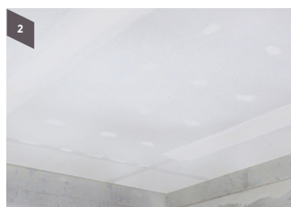
Step 2 Start in one corner and work progressively across the ceiling
