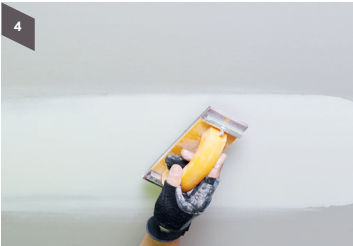
Step 4 When compound is dry, lightly sand at 45 degree with a sanding block
