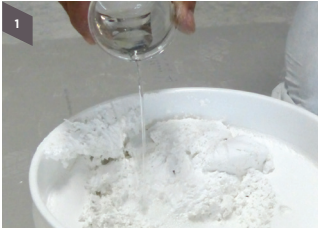
Step 1 Check the consistency of the Mac Plaster Spray Applied Finish
