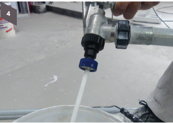
Step 4 Two coats of Monosilent Spray Applied Finish must be applied
