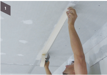
Step 1 Fill in the joints with Monosilent compound
