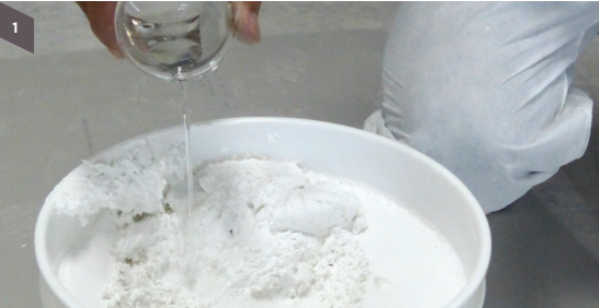
Step 1 Check the consistency of the Monosilent Spray Applied Finish
