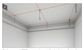
Fix hangers at 1200 mm o.c in a gradient scheme above the lines of primary channels  $\,$
