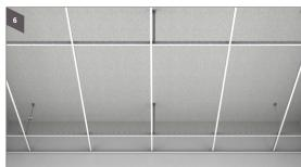
Insert the long cross tee to main tee in place for  $600 \text{x} 600 \,$  module
