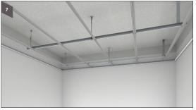
Connect the spring tee to the primary channel at 600 spacing Insert the clip in panel to the exposed spring tee using wire connecting clip WCC
