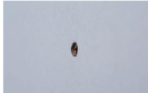
*Poor fixing of screw into plasterboard*
