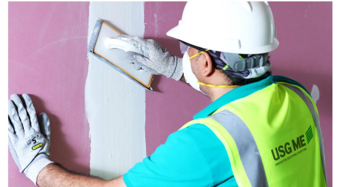
*Application of joint compound over tapered edge joint*
