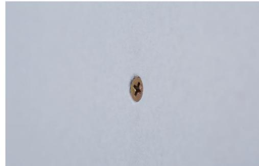
*Good fixing of screw or fastener into plasterboard*
