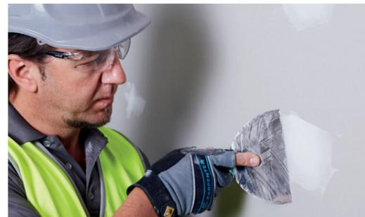
**Applying 3 separate coats of joint compound over screw fixings**
