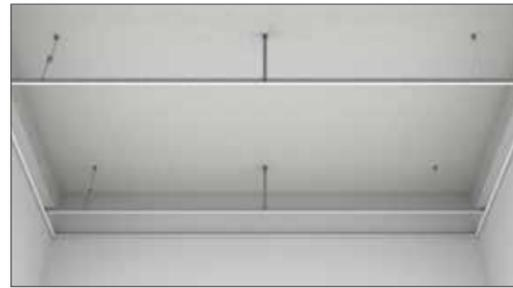
Fix the main tee at 1200 mm spacing and lay it on the wall angle.
