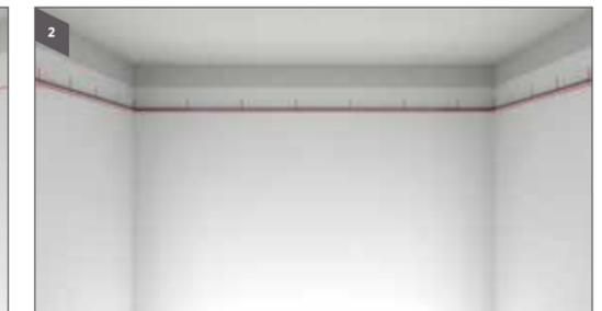
2 Install wall angles around the perimeter at marked locations using screws at 450 mm o.c
