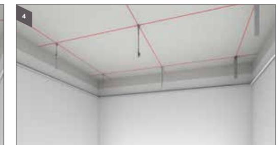
4 Fix hangers at 1200 mm o.c in a gradient scheme above the lines of wall angle
