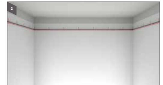
Install wall angles around the perimeter at marked locations using screws at 450 mm o.c
